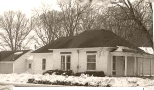
Harriet K's Cottage before renovation
